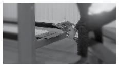
4 Lever the platform out towards the posts using a metal pole (or other sturdy lever) until there is enough space to fit the Air Jacking Beam between the platforms.
